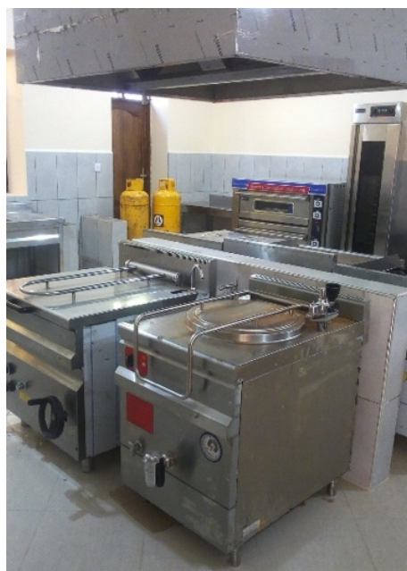
Figure 14: New kitchen in Mvimwa
